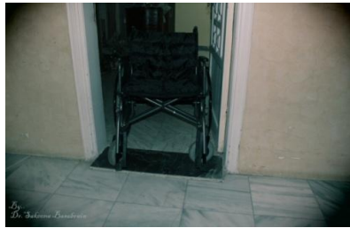
Fig. 3. Available space for the movement of the chair is not flexible enough for the passage of the chair easily by threshold and increase the difficulty of Use
