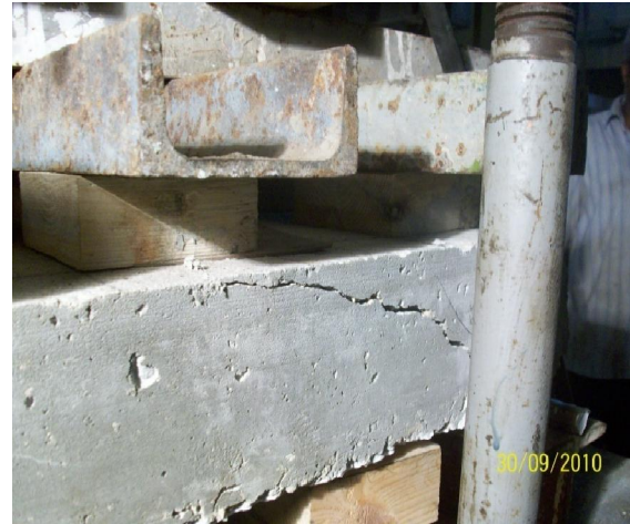
Figure (4): Shear failure of slab S1
