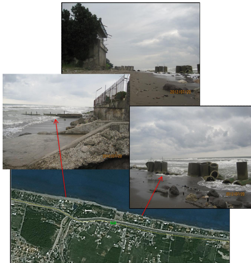
Fig 6. Destroyed buildings in expose of sea waves in Sisaraa coast
